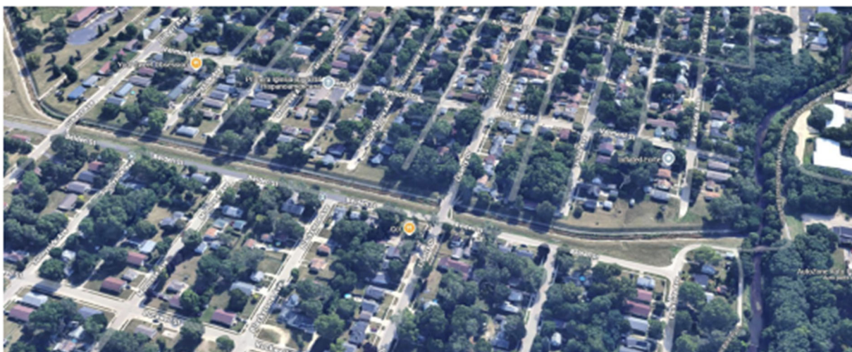
Figure 1: Aerial view of concrete channel in Beverly Park neighborhood
